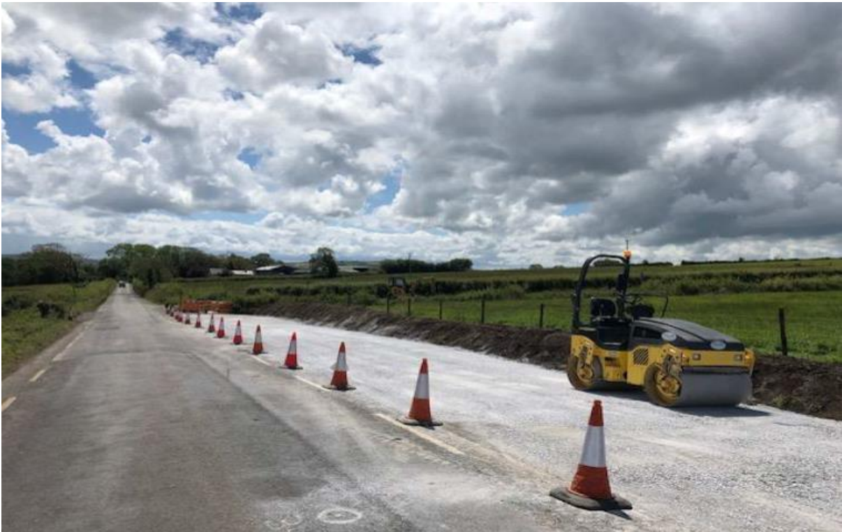
Image 4.16: Example of Passing Bay Construction
