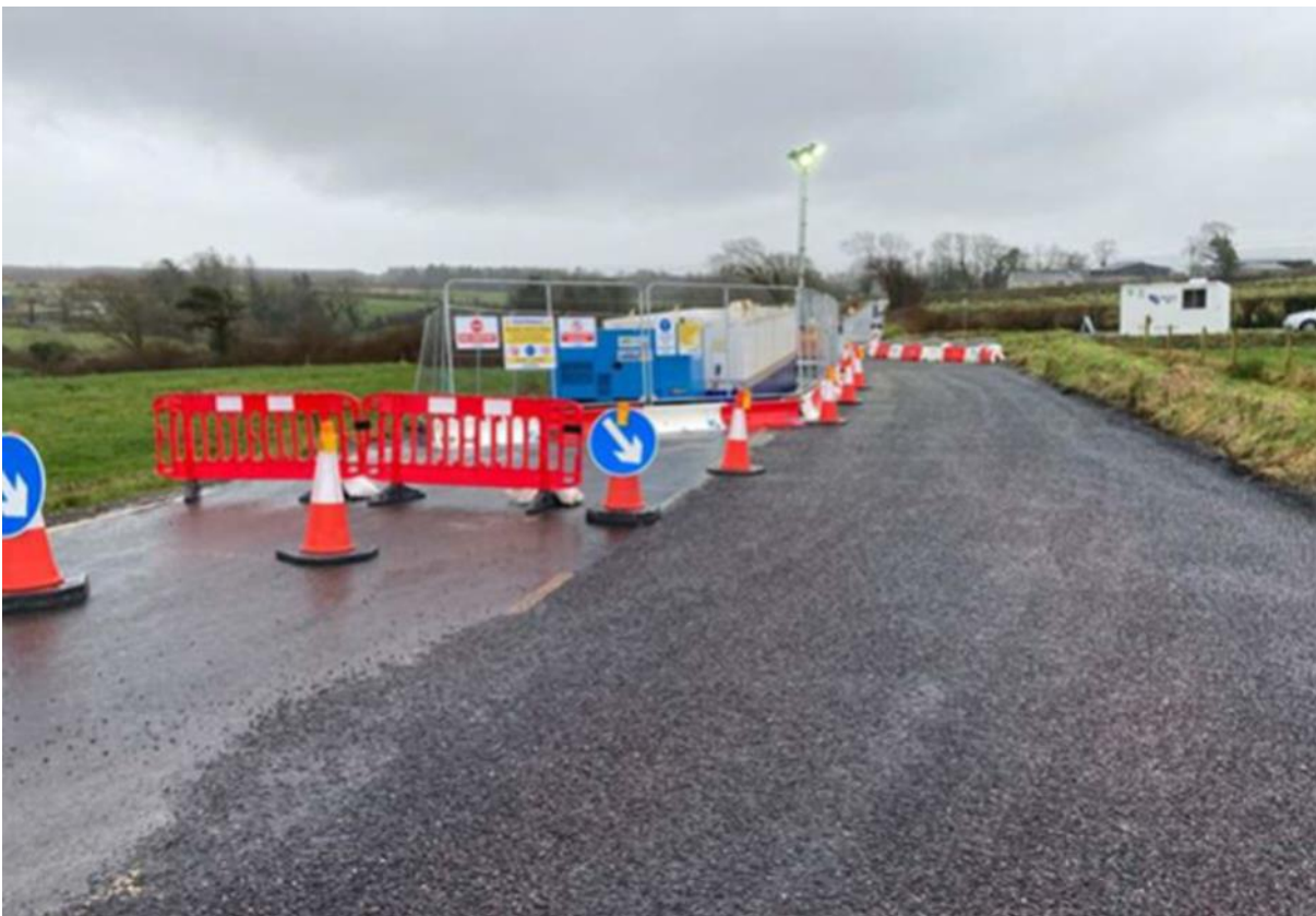
Image 4.17: Example of an Operational Passing Bay with Joint Bay under Construction
