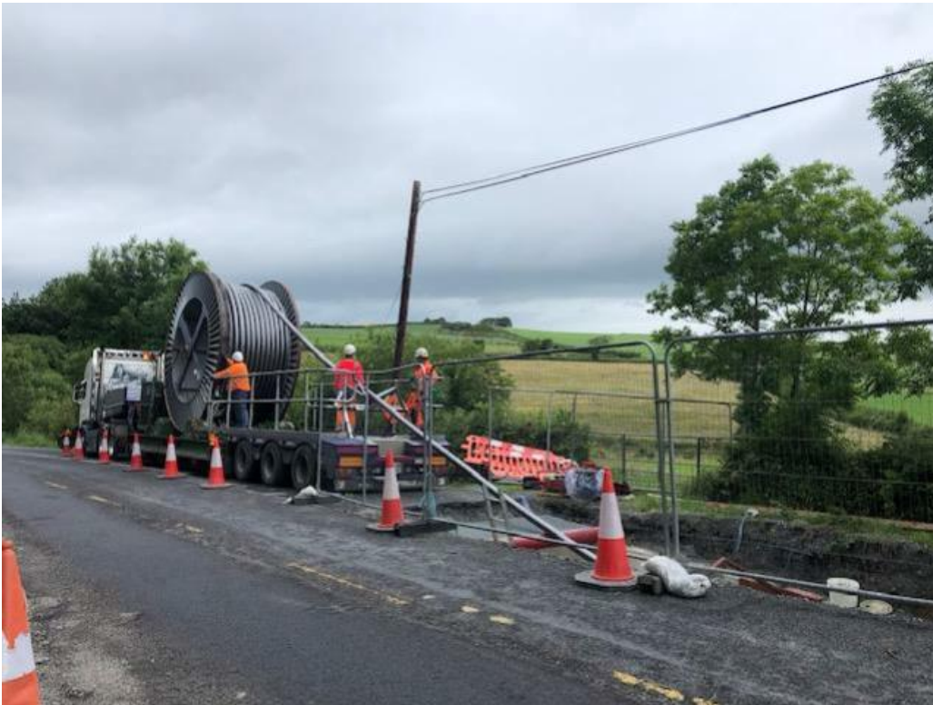
Image 4.23: Example of a Cable Pulling at a Joint Bay
