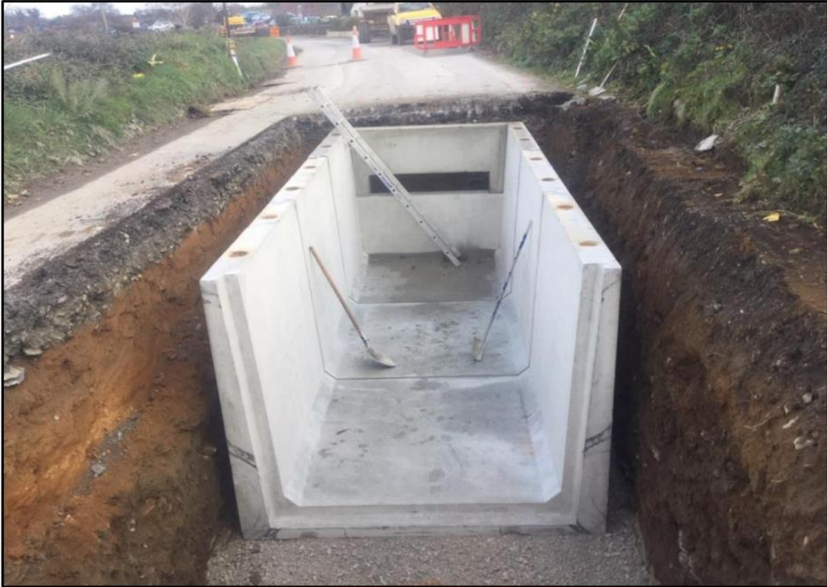
Image 4.2: Example of a Joint Bay During Construction
