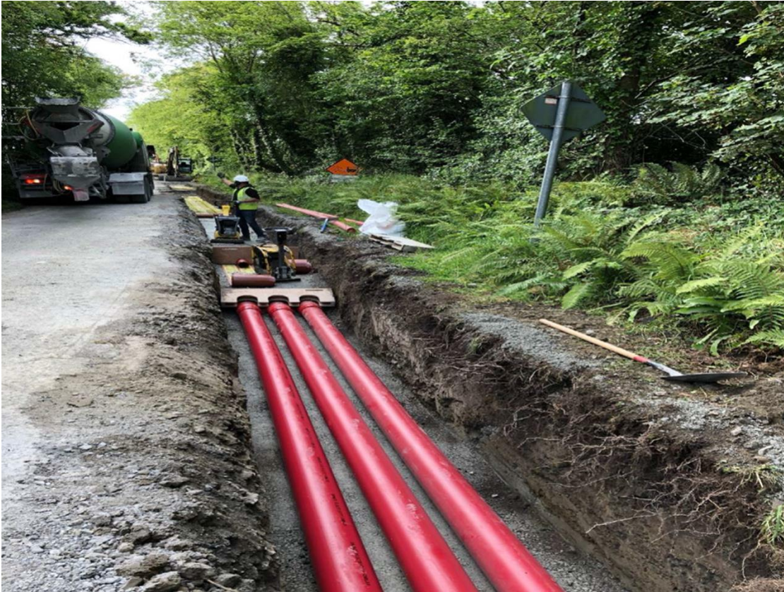
Image 4.12: Example of a Cable Trench In-Road with Cables in Flat Formation
