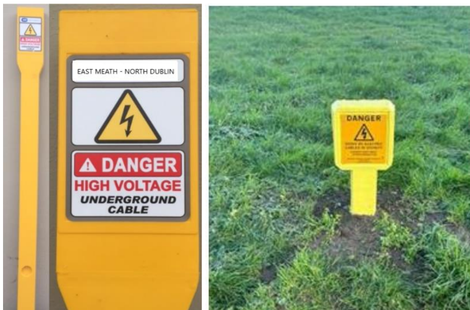
Image 4.18: Examples of an Above-Ground Cable Route Marker Post
