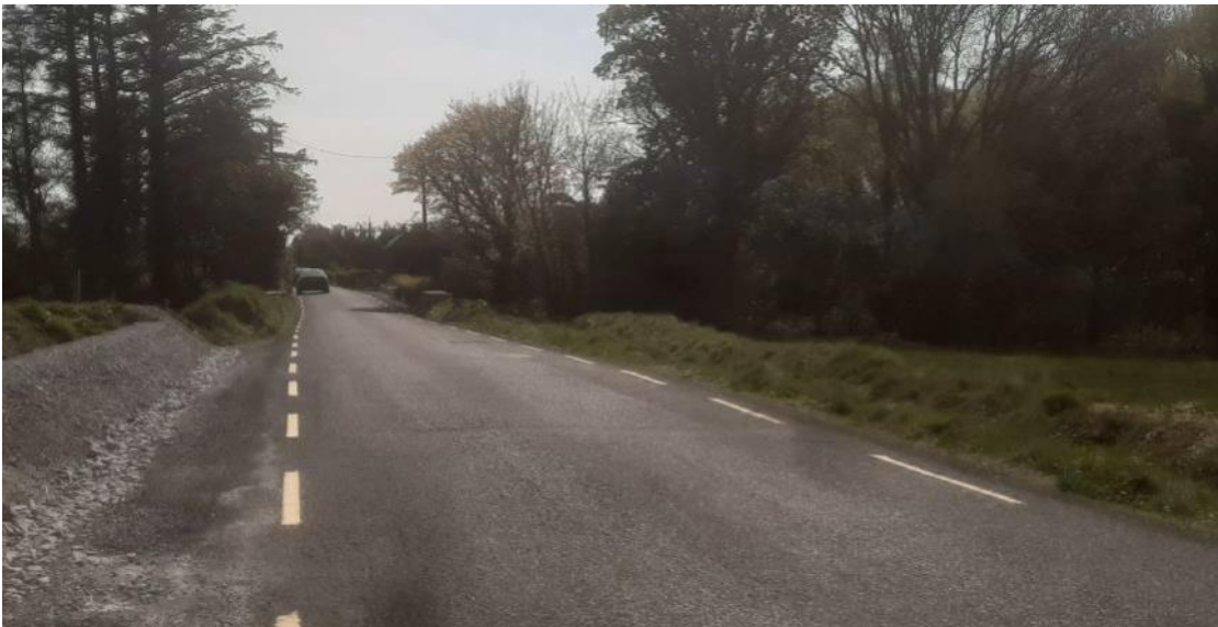
Image 4.13: Example of a Reinstated Road Following the Laying of Underground Cables
