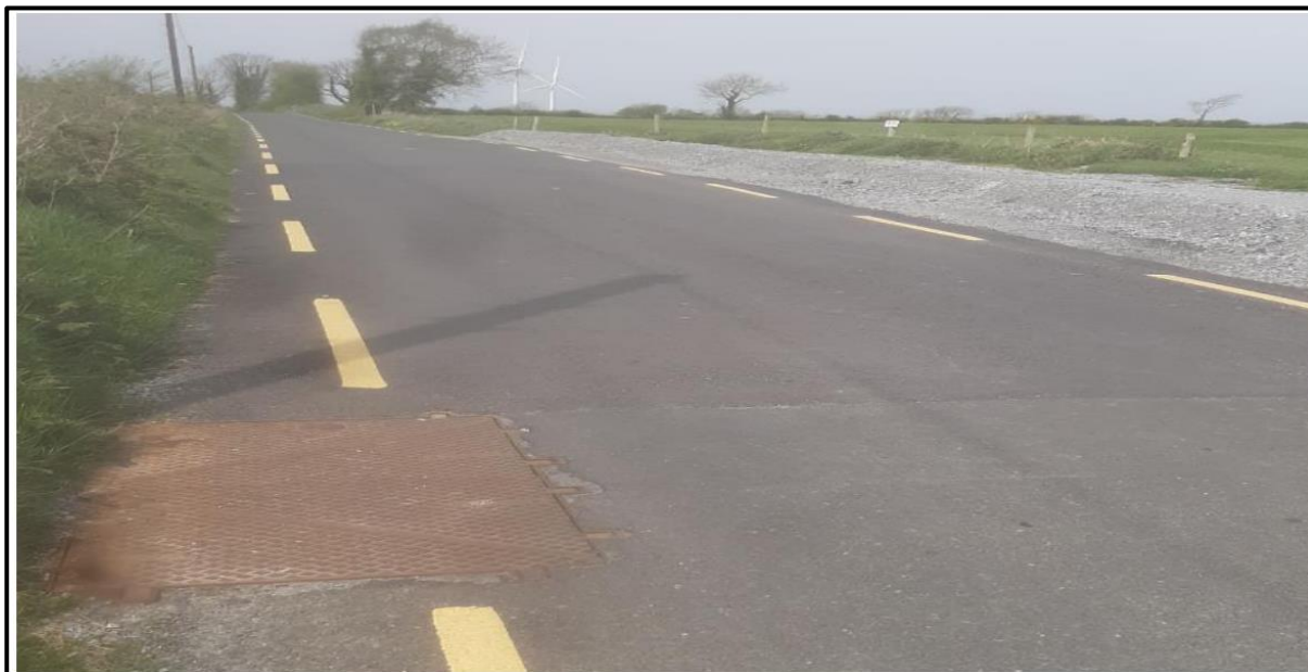
Image 4.3: Example of a Reinstated Road Over a Joint Bay (Darker Asphalt) with the C2 Chamber Cover Visible
